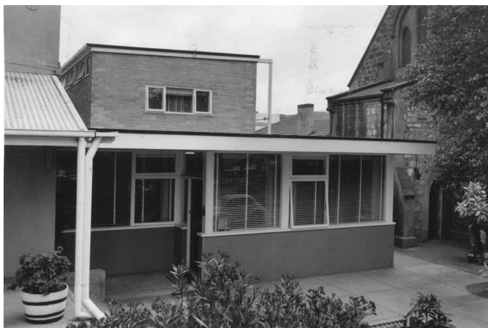
New offices and C.B. Howard Hall, with flat above, opened 1960. Photo Don Gee.
