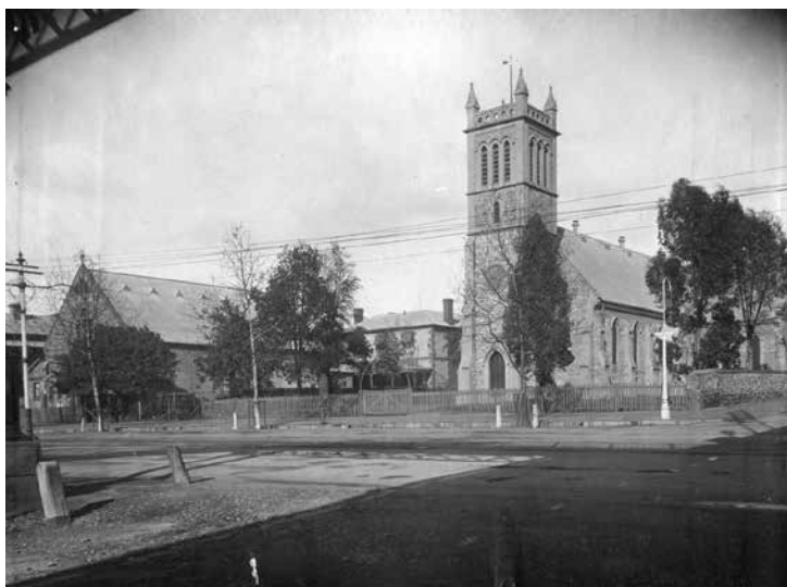
Trinity church after the 1888 rebuild with the rectory and 1880 parish hall, and with established trees. The old Morphett Street bridge structure can be glimpsed above.
