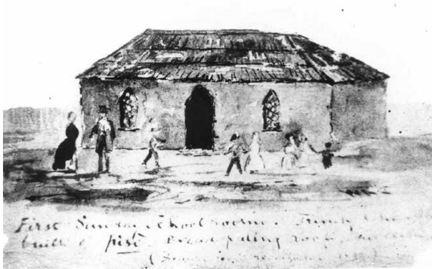
The first Sunday school room, built in 1839 of pise and the residue of the unusable pre-fabricated church. SLSA B8042. author unknown.
