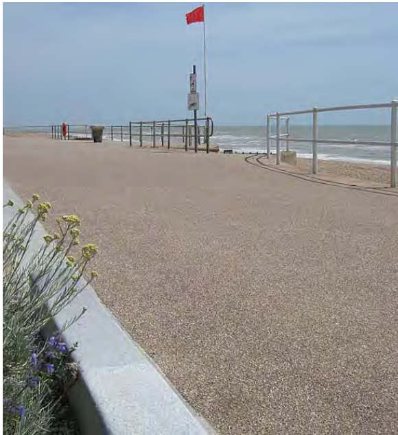
Resin Bonded Gravel on pathways
