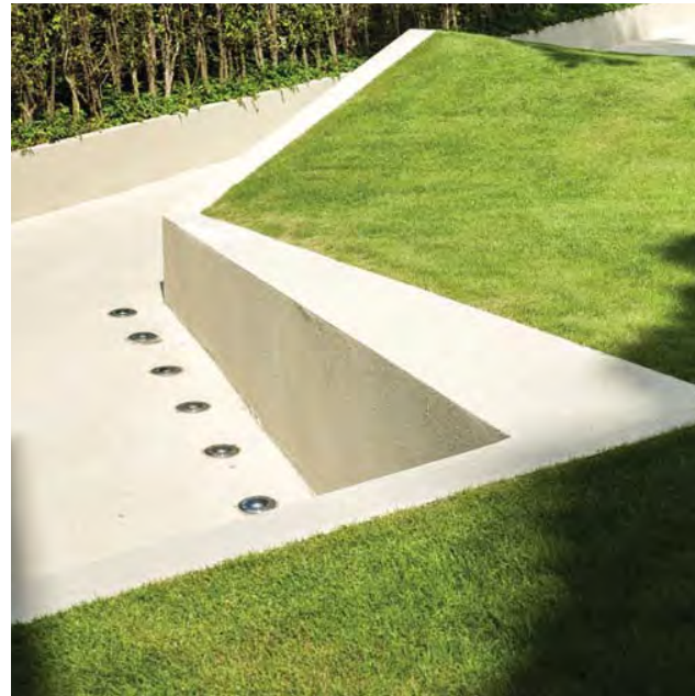
Bespoke Concrete Planter & Seating Edge (Part of Permanent Works)
