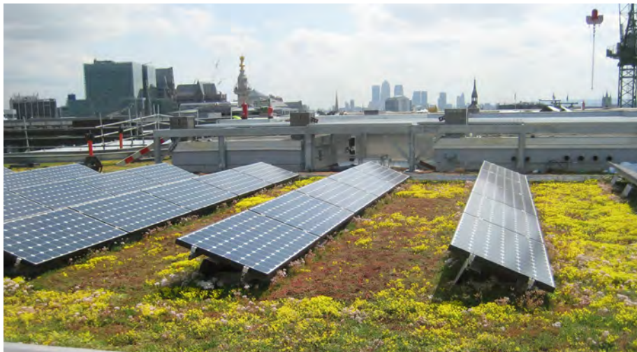
Watermark Place, London Solar pannels intergrated with sedum planting
