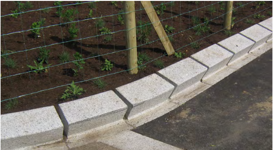
SUDS Cuts in raised kerbs can allow surface water to run into planted areas.
