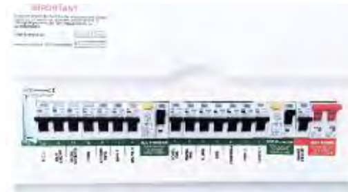
Utility Cupboard Consumer Unit
