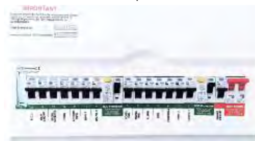
Utility Cupboard Consumer Unit
