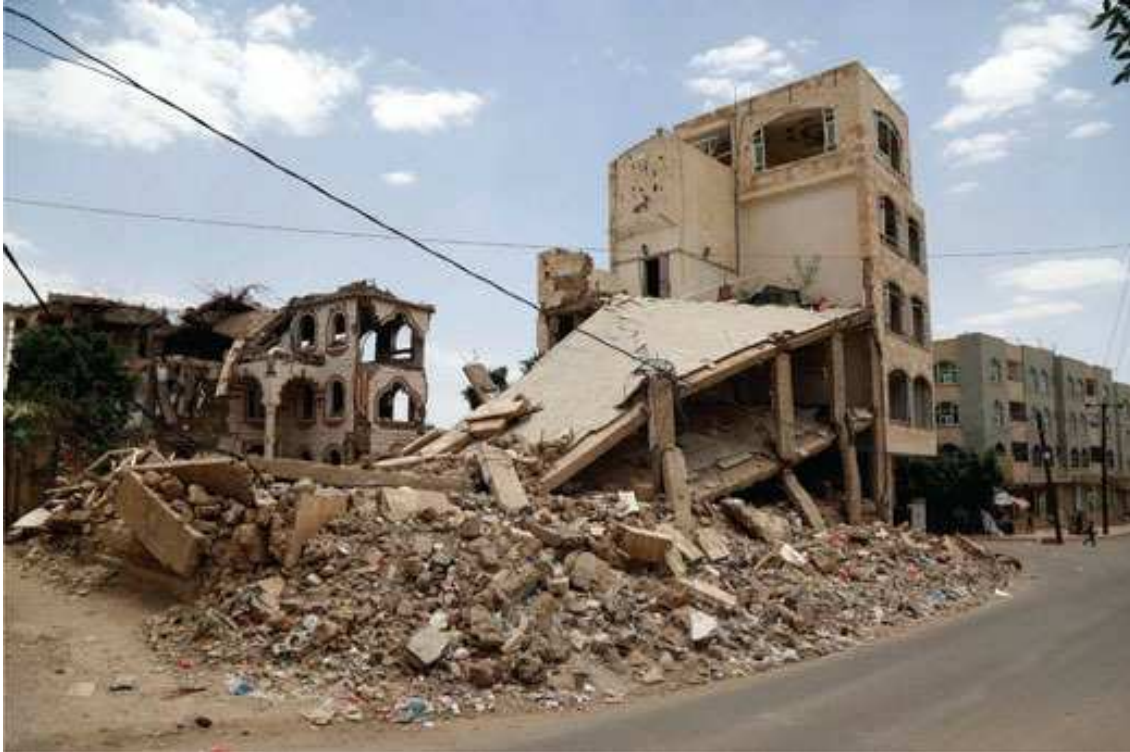
Plate 4.2 Destroyed buildings, Sana'a, Yemen, June 2019
