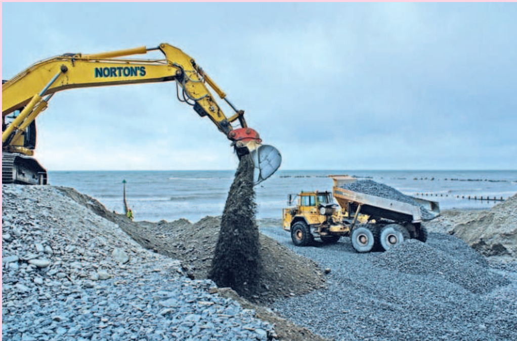
Plate 3.2 The building of new flood defences on Borth Beach, Wales, UK
