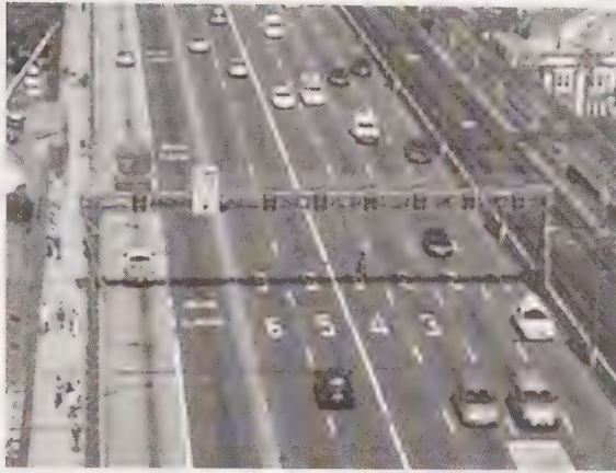
Figure 14.2 Lane-marking gantries on the Sydney Harbour Bridge
