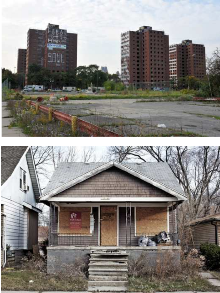
Figure 3.8 Abandoned residential buildings in Detroit, USA
