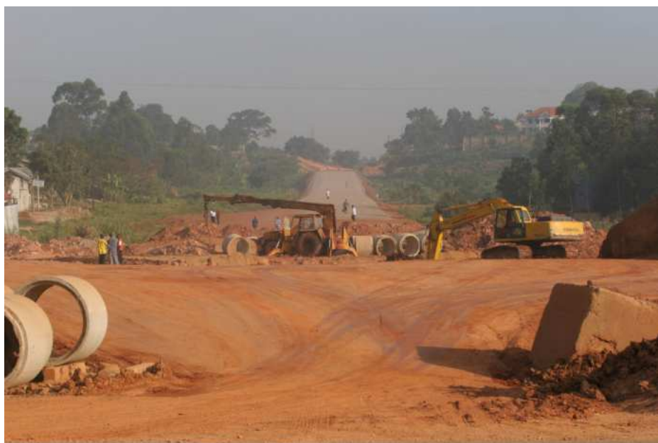
Figure 10.1 Construction work along the road from Kamwenge to Fort Portal in western Uganda
