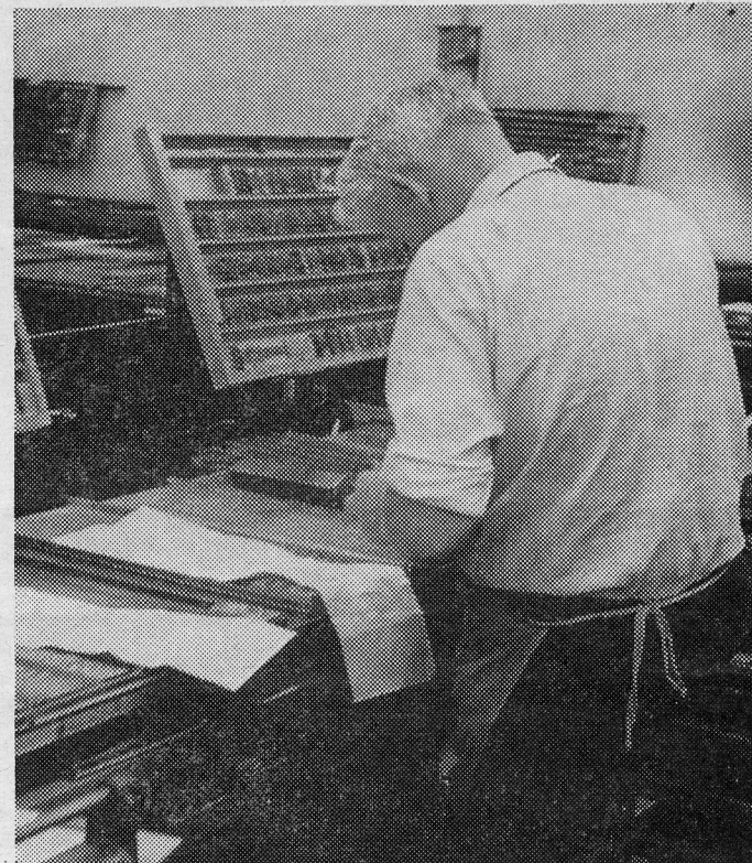
ABOVE: One of the machines that transforms photos into printing blocks.
