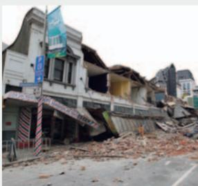
Sections of the city, including the city's landmark Christchurch Cathedral have been damaged. Christchurch is built on silt, sand and gravel with a water table lying directly underneath the city. This makes the city particularly vulnerable to the process of liquefaction of the soil during an earthquake.
