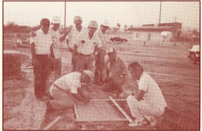
Putting our name in concrete. John Sunahara, Mas Sunahara, Jim Kobata, Duke Takeuchi, Ted Kobata, Sid Arase, Jim Namba and Sus Satow.
