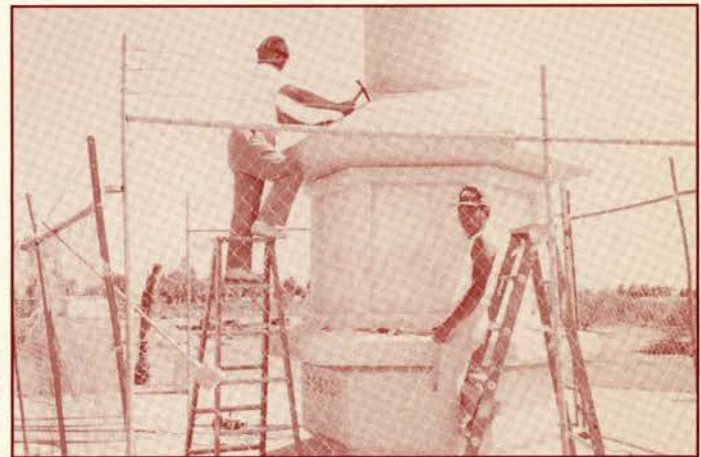
Two Georges, Oki and Yomogida, put finishing touches with chipping hammers.
