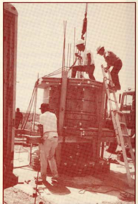
Monument form in place. Ted inspects for true position with Sid Arase.
