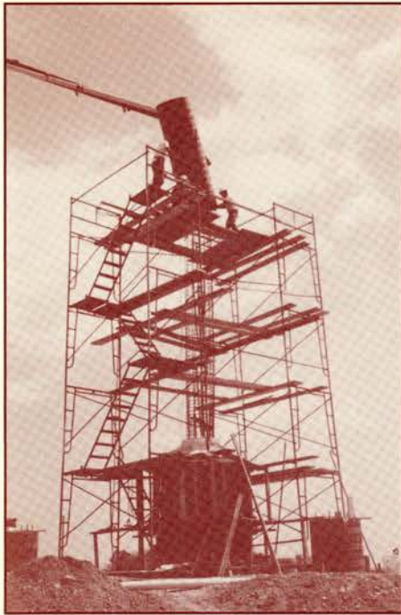
Installation of the 3 ft. diameter sauna tube form.
