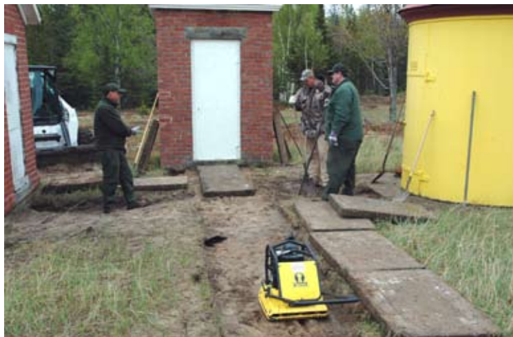
Sidewalk and landscape work
