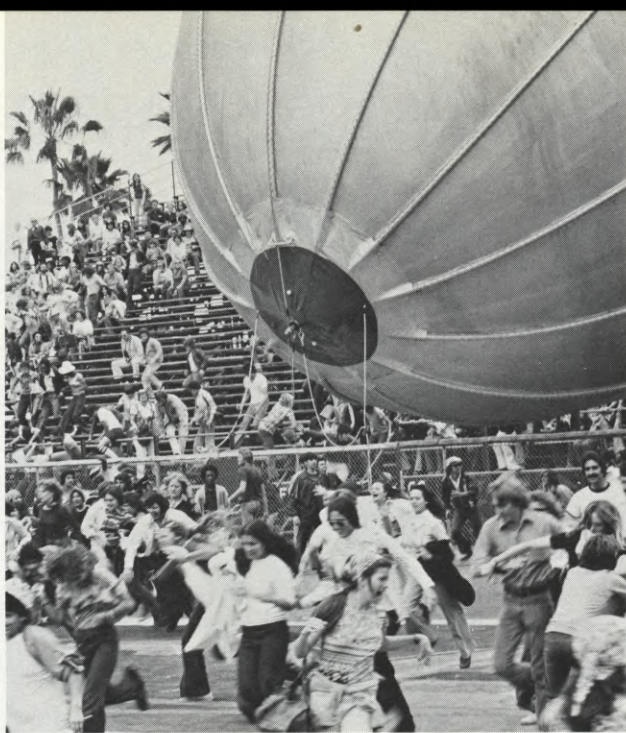
(LEFT) The 40-foot blimp mock-up shown against a front projection background plate of Miami Stadium crowd fleeing in panic. (RIGHT) Plate shot of the same action at the same time, but from a higher angle, is used to film a blimp interior with Bruce Dern in the foreground. The front projection system permits compositing of intricate effects, with the complete scene being available for screening the next day.
