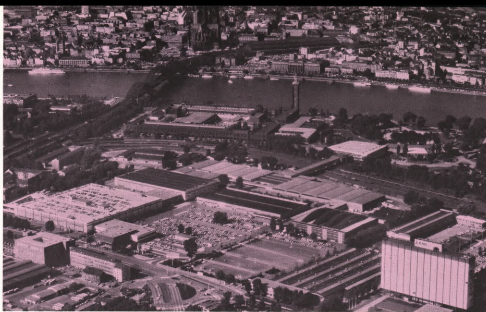
The enormous complex of twelve exhibition halls on the banks of the Rhine River which, every two years, is the site of Photokina , the World Fair of Photography. In the background (top) can be seen the famous Cologne Cathedral, spectacular landmark of the city, and a familiar site to those visiting the many trade fairs and exhibitions held in Cologne.
