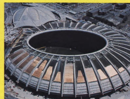
(LEFT and CENTER) Three-dimensional architectural models of the Olympic Park sports complex as it will look when completed. The rakish Tower will support, by means of cables, a retractable "lid" that will protect the field in inclement weather, but leave it open to the sky when the weather is fair. (RIGHT) The Olympic Stadium under construction. (BELOW) A three-dimensional model (LEFT) and two actual views of the Olympic village with its striking "half-pyramid" structures.
