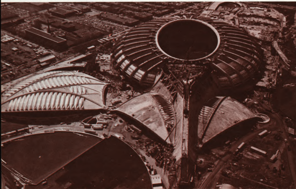
An aerial view of the fantastic sports complex at Olympic Park in Montreal, shot on May 6, 1976, scarcely more than two months before the start of the Games. The upper structure of the tower and the amazing retractable "lid" did not get finished in time, but a final super-human effort completed the really necessary facilities. Montrealers, highly critical of the huge cost overrun before the Games, loved their magnificent Stadium once it became a reality.
