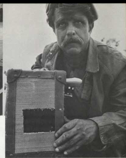
In an effort to get spontaneous action of the extras "living" in the migrant camp built for the film near Stockton, California, an Arriflex 35BL camera was installed in a suitcase with a port hole cut into the end. The camera operator, dressed to match the extras, was able to move inconspicuously among them and film their unstudied reactions. This lent an additional documentary touch to the sequence.
