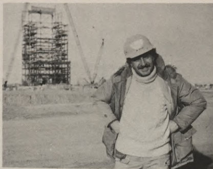
Director Mel London of Vision Associates standing in front of construction site of a new coal-fired power plant in Emory, Utah.
