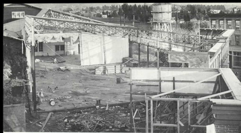
(ABOVE) The William Fox Studio, 1918, formerly the Thomas Dixon Studio, located at Western Avenue and Sunset Boulevard. It later became an auxiliary facility of 20th Century-Fox Studios. (BELOW) Previously (1917) the William Fox Studio had temporarily been housed at 1845 Allessandro St., the old Selig Studio in Edendale.
