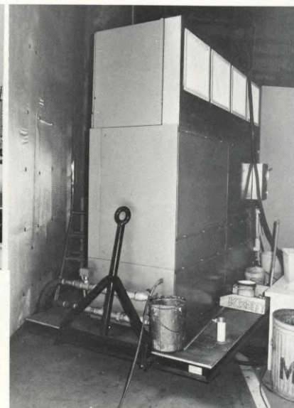
Although heating has been provided inside the stages, the refrigeration units for air conditioning are portable and placed outside the stage. These units (101) supply cold water which feeds into the stage through accessory holes. (RIGHT) Cold air blowing unit, which is fed cold water from refrigeration unit outside the stage.
