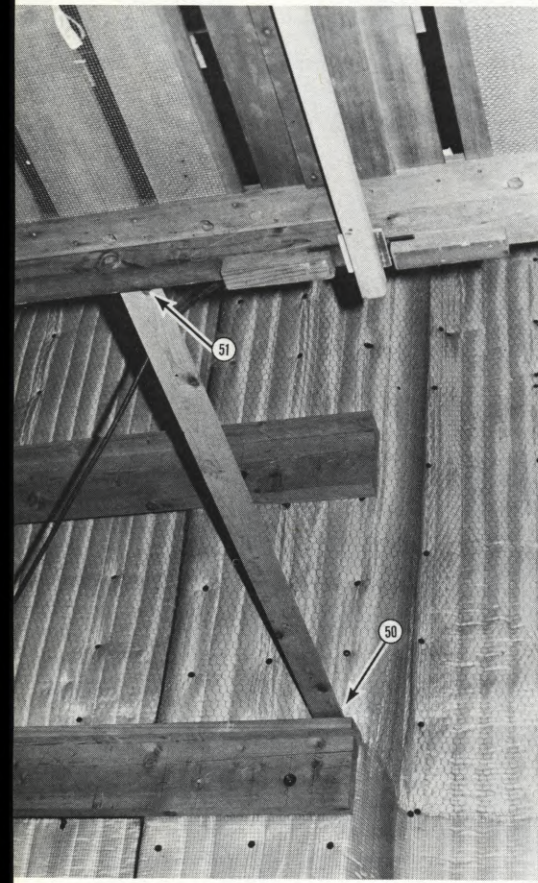
(ABOVE LEFT) The brace nailed to the wooden batten (50), which is mounted on the walls and connected to a parallel. (BELOW LEFT) The catwalk system at grid level has gates which allow for safe access around the entire stage grid. (1) One of the pair of double doors at grid level connecting the two stages. (2) receptical for A.C. auxiliary power. (3) Bus-duct system for distribution of electrical power. (RIGHT) Each stage has a large access area with rail and jib crane for convenient lifting of heavy loads from floor to grid.
