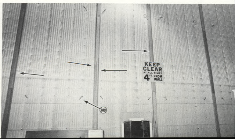
(LEFT) A corner of the stage, showing on-stage dressing rooms, a set rigged with lighting, and the overhead grid structure. (RIGHT) This wall is removable, so that the two 14,000-foot stages can be expanded to a single 28,000-foot stage. Each removable section is approximately 10 feet wide and 35 feet high. Despite the height and sound integrity of these removable sections, they are relatively light in weight and can be removed quickly with the use of a crane. (100) lifting lug used to hoist sections.
