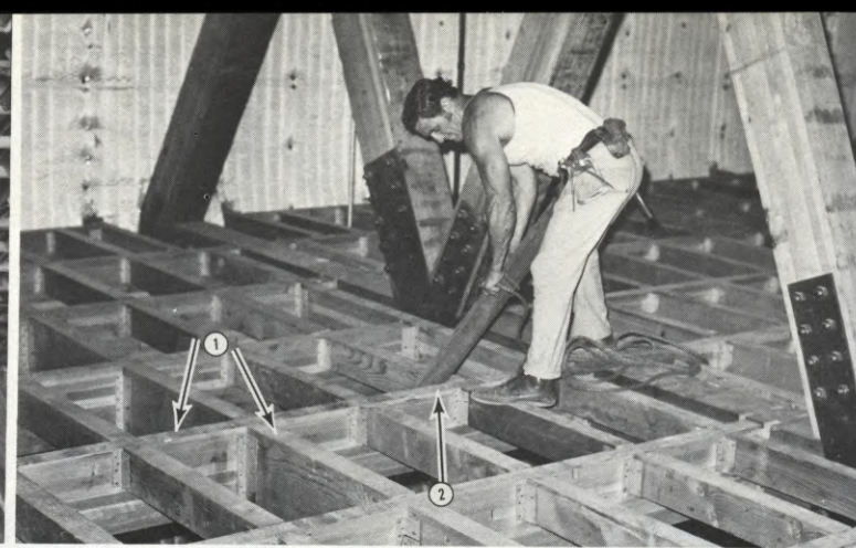
(LEFT) An area of the overhead grid, which is 35 feet above the floor level. Wooden braces can be conveniently nailed to all members of the wooden grid. Arrow points to very long brace used to secure parallels. (RIGHT) View showing how wooden braces can be brought through grid and nailed to any of the grid members. Design provides for every member to carry maximum load. Openings are small enough to insure safety of man walking on grid, but large enough to permit any type of brace to be used through it.
