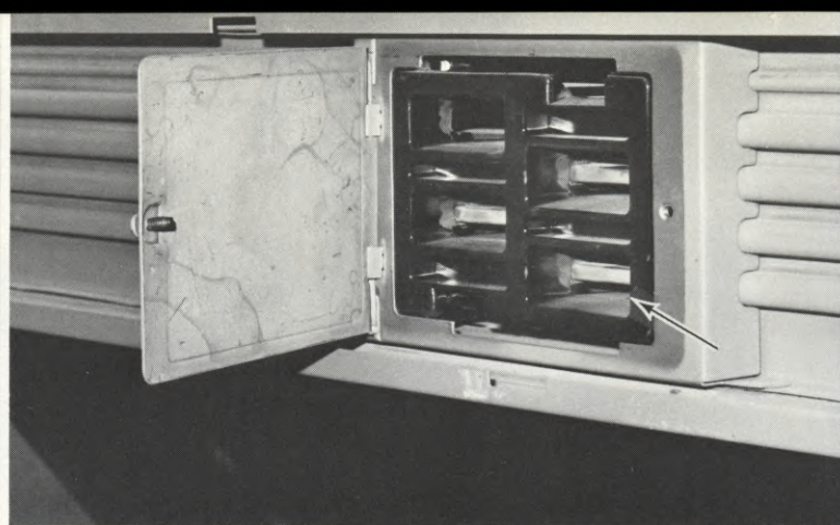
(LEFT) Detail of the bus-duct system installed on the grid level along the catwalk. (10) the bus-duct system itself; (11) contactor box, which connects directly to the bus-duct; (12) the safety door which covers the connector box. These connector boxes are conveniently located on 24-inch center contactors. (RIGHT) Detail of the connector box, which is part of the bus-duct and which allows standard stage plugs to be directly connected to the main power.
