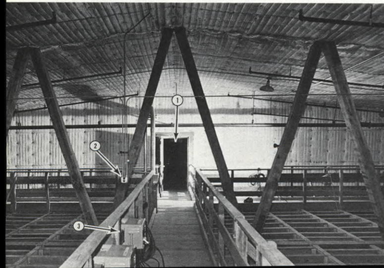
(ABOVE LEFT) The brace nailed to the wooden batten (50), which is mounted on the walls and connected to a parallel. (BELOW LEFT) The catwalk system at grid level has gates which allow for safe access around the entire stage grid. (1) One of the pair of double doors at grid level connecting the two stages. (2) receptical for A.C. auxiliary power. (3) Bus-duct system for distribution of electrical power. (RIGHT) Each stage has a large access area with rail and jib crane for convenient lifting of heavy loads from floor to grid.
