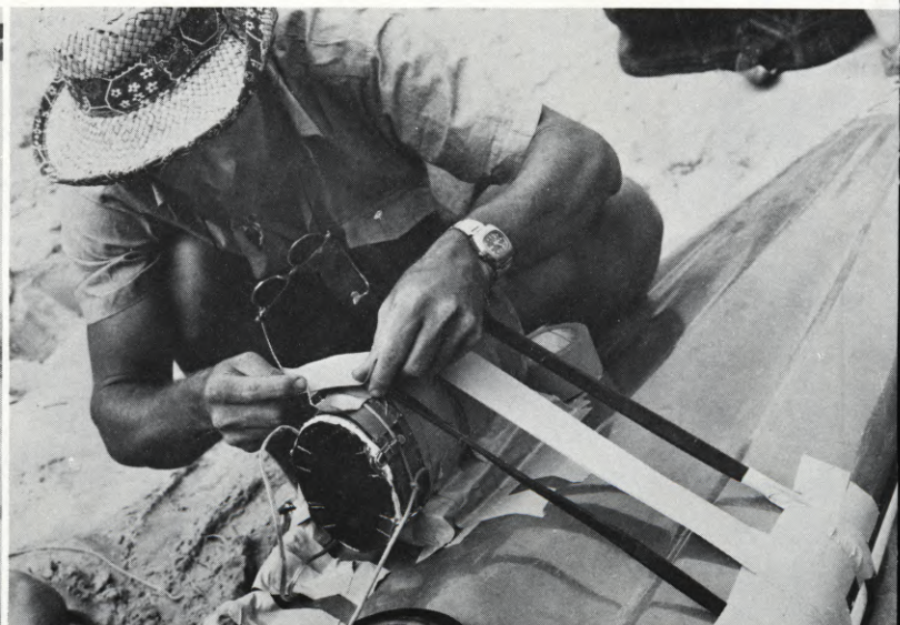
(LEFT) Walt Blackadar and Fletcher Anderson discuss the "hydrodynamics" of the GZAP camera, as mounted on the front of the kayak. This camera proved ideal for filming kayaker's point-of-view shots, because it is so light in weight and does not make the boat harder to run when it is mounted. A 10mm lens on the camera, mounted as shown here, very closely duplicates what the kayaker sees when he is on the water. (RIGHT) The camera mount is attached to the kayak by means of a combination of shock cord and gaffer tape. (ABOVE RIGHT) Roger Brown readies the Milliken high-speed camera for shooting at Lava Falls.
