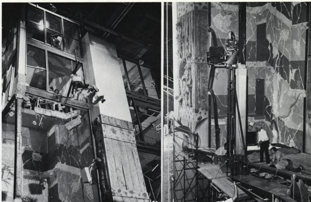
(LEFT) Stuntmen jump from the top of a 50-foot structure, representing the upper floors of a 25-story skyscraper. The set was built of structural steel on Universal's Stage 12, after a 20-foot pit had been dug in the floor. (RIGHT) The camera, on a crane, moves into the set.
