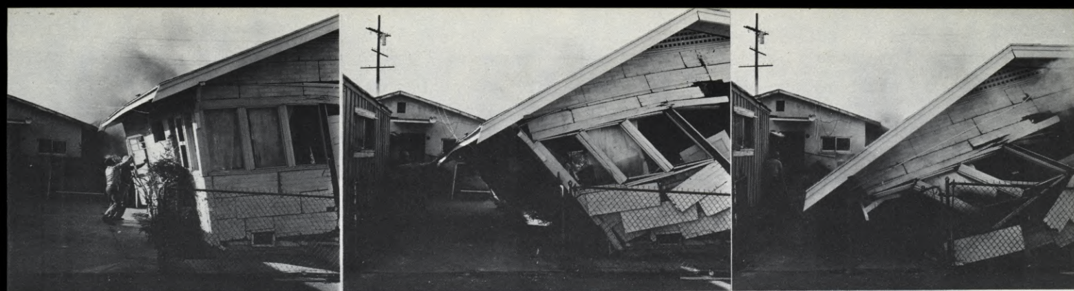
A small house topples and collapses. Breakaway construction of the building was designed by Art Directors, but the rigging for destruction was worked out by expert riggers of the special mechanical effects team. The effect shown here was relatively simple to prepare, but some of the more complex effects required four or five days to rig, with the rigging crew constantly working ahead of the shooting schedule.
