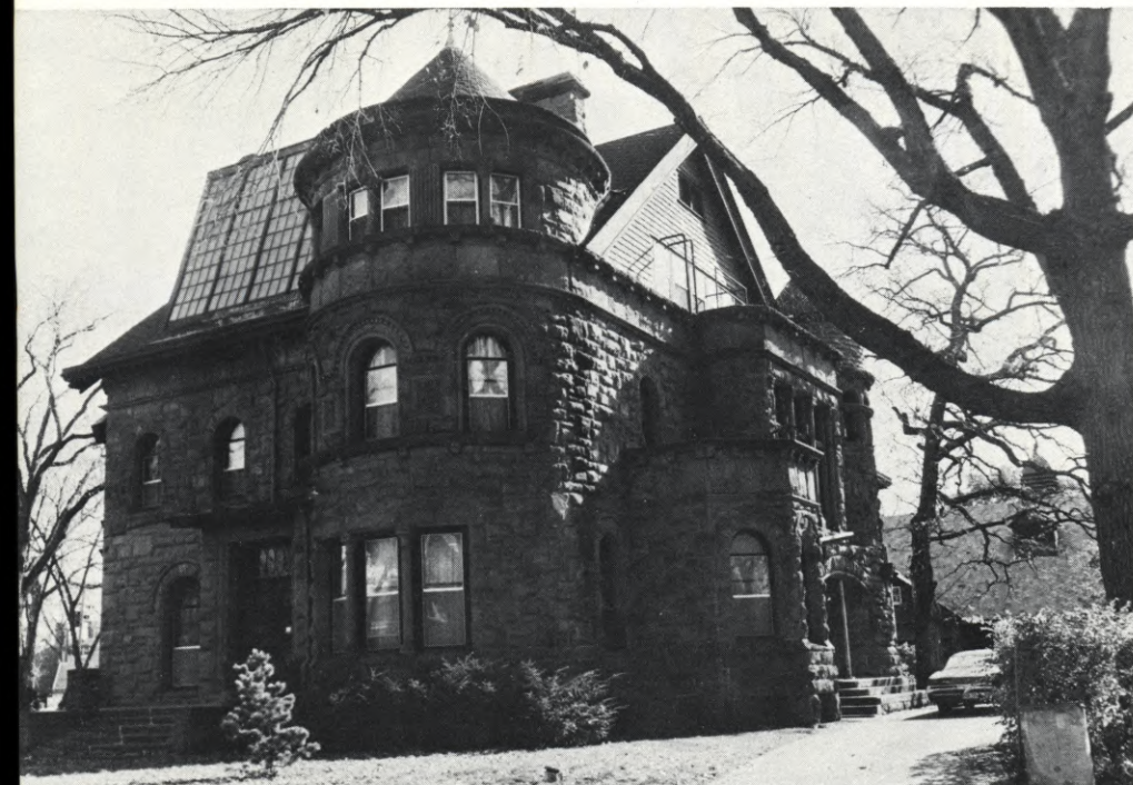
The house in St. Paul that Carl Weschke and his family live in, and which also houses Llewellyn Publishing Co., is a spooky old brownstone mansion, haunted by the ghost of a suicide servant girl. It is here that the rituals of Weschke's coven are conducted. "A perfect pad for a witch," says the enthralled author.
