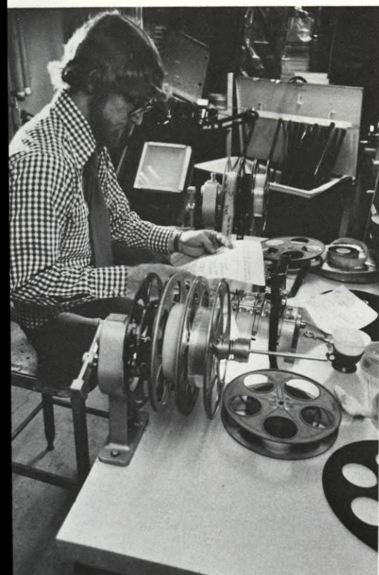
(LEFT) Film editor Todd Martin lines up 35mm anamorphic print-downs of the 70mm footage used in cutting. (CENTER) A modified old-style projection Moviola turned on its side solved the cutting problem, turning the image upright on the viewing screen. It worked well enough, but occasionally punched its own extra set of perforations in the 35mm squeezed dailies. (RIGHT) A close look at "precision detailing" of the 2" x 4" cradle which held the Moviola in position for vertical viewing.
