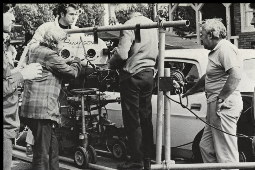
(LEFT) Panavision camera mounted on miniature dolly set up on outrigger platform alongside the car. (RIGHT) Keach, suspended from the force, walks with friend, while camera dollied in front of them. Old trick of dollying light-weight Brute, plus spot/flood, minimizes travel and keeps lights out of the camera angle. Camera "holds size" on couple with zoom lens, and also makes lateral dolly move for perspective change past poles and trees.
