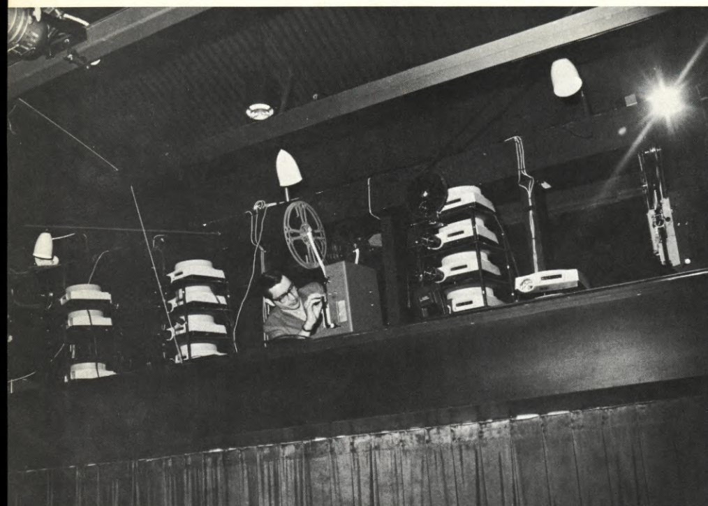
Projection booth in San Francisco's Electrovision theatre houses 29 Kodak projectors—three 16mm Pageant movie and 26 Ektagraphic slide projectors—linked by a computer into a multi-media marriage of sight and sound. Each performance is activated by the push of a single button which controls not only the visuals and sound, but special effects and house lights.
