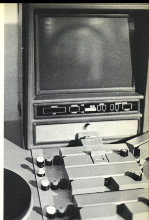
Large, bright screen and advanced picture-sound quality enable the Moviola Console to be used as a "preview theatre", as well as an editing device.
