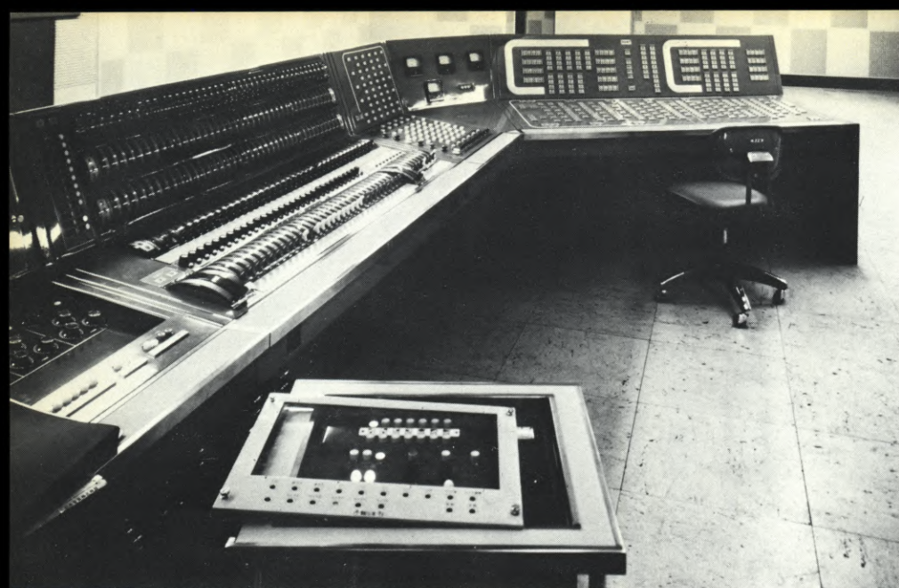
Each color television stage of the NHK complex has its own huge control console for handling the totally automated lighting on the stage. Controls include raising and lowering of individual units, spotting or flooding the beam, panning and tilting and automatic changing of color filters.
