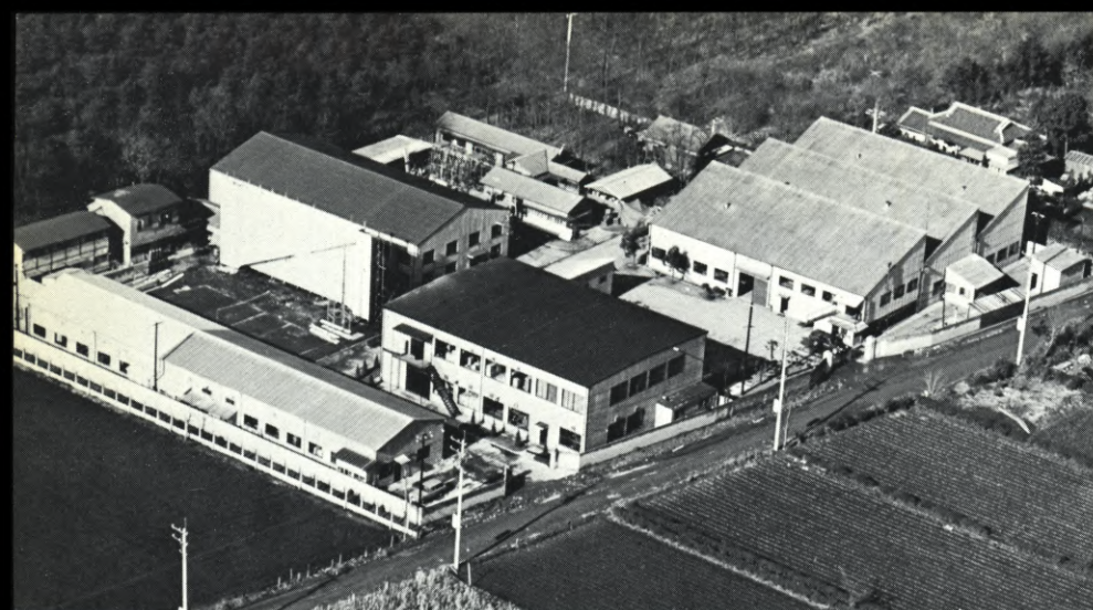
The main factory complex of RYU-DEN-SHA & CO., LTD., (Ryu Electric Company), focal point of the Asian lighting industry, as seen from the air.
