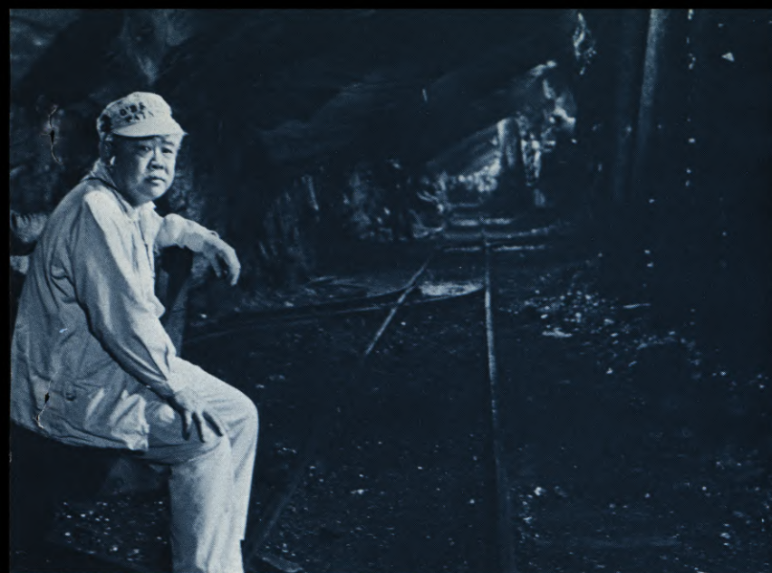
(LEFT) Cinematographer Howe, clad in white "dust suit" to protect his clothes, surveys incredible coal-mine "set" stretching 400 feet through Paramount Stages 12, 14 and 15. Massive construction was an exact reproduction of an actual mine created by Art Director Tambi Larsen using 138 plaster casts of the mine walls. (RIGHT) The Hollywood coal-mine ready for a take, lighted with concealed quartz lights.
