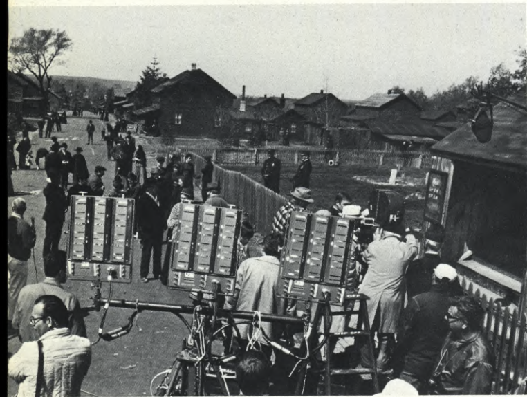
(LEFT) Shooting down the main street of Eckley, Pa., the only "coal patch town" in America that exists almost as it did a century ago. In the foreground are three Berkey/Colortran Mini-Brute luminaires, each accommodating nine PAR 36 tungsten-halogen lamps. (RIGHT) A bank of quartz-cluster units lights up location exterior on an overcast day. Such units completely replaced cumbersome arc lights formerly considered absolutely essential on a feature of so vast a scope.
