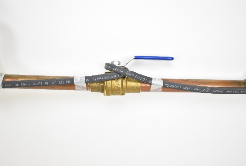
FIGURE C Connect cable to pipe and tape (step 6).
