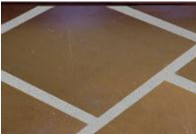
Fiberboard with Seams Taped
