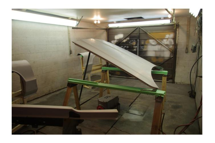
Getting set up to shoot the black. I bolted the hood hinges to saw horses and propped it up so I could paint both sides in the same shoot.
